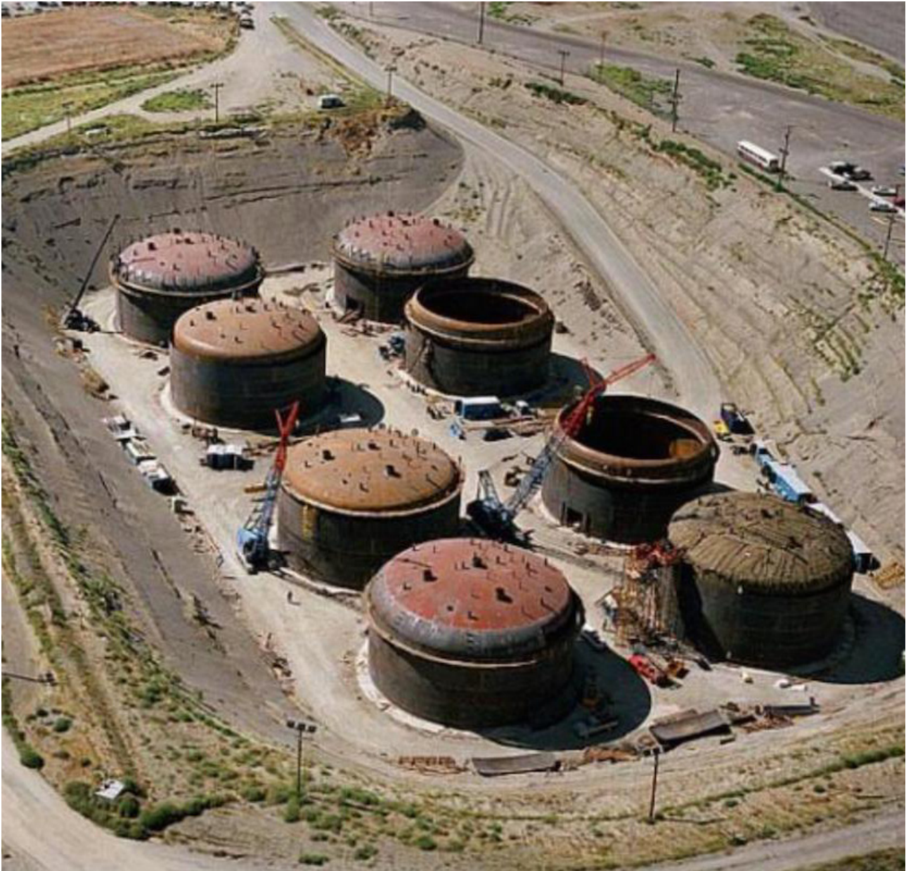
► Figure 18. Reconstruction of the tank farm for storing strategic fuel reserves for the Regional Force Grouping. Pochinok, Smolensk Region
